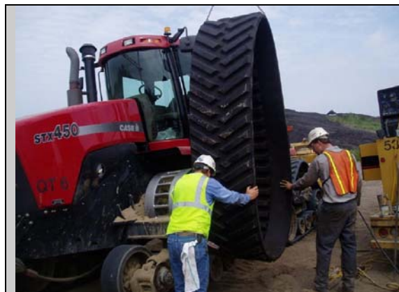
Using a boom truck to remove track
